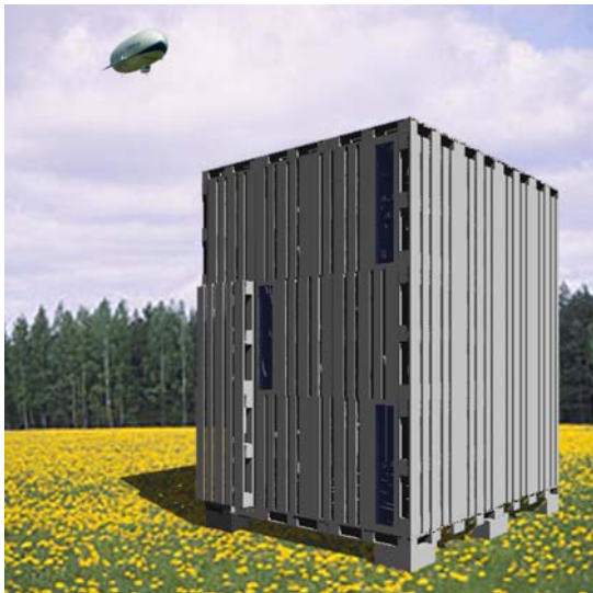
Figure10: Framing of PHS© Pallfrigggebod in Sweden. This elemental dwelling can be raised in any plot not exceeding the layout plan 10 m 2 . Source: Suau.
