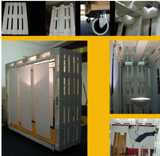
Figure 4: Constructive test of PHS-F1© developed in Sweden. After several simulations, the adopted connector system is based on galvanised gang-nail punched metal plate fastener; wood screws and round wire nails. The roof is supported by a tensile V-
