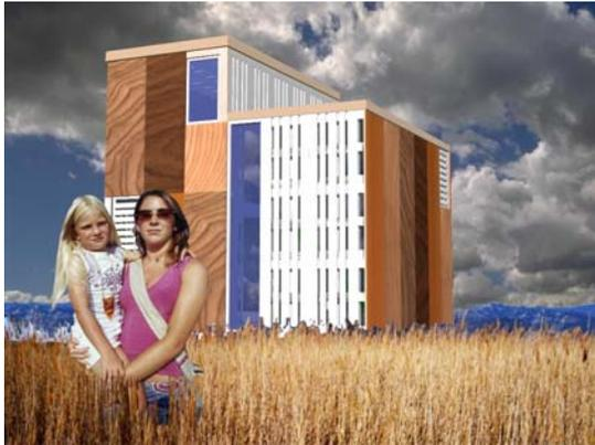
**Figure 7:** Rendering of PHS© Mediterranean case, outskirts of Barcelona (nearby Cerdanyola). The structure consists of a Euro-pallet frame, based on 120cm times 80cm each board. It is oriented to south and has double skin. The outer envelope towards south is a whitened shading device. Source: Suau.
